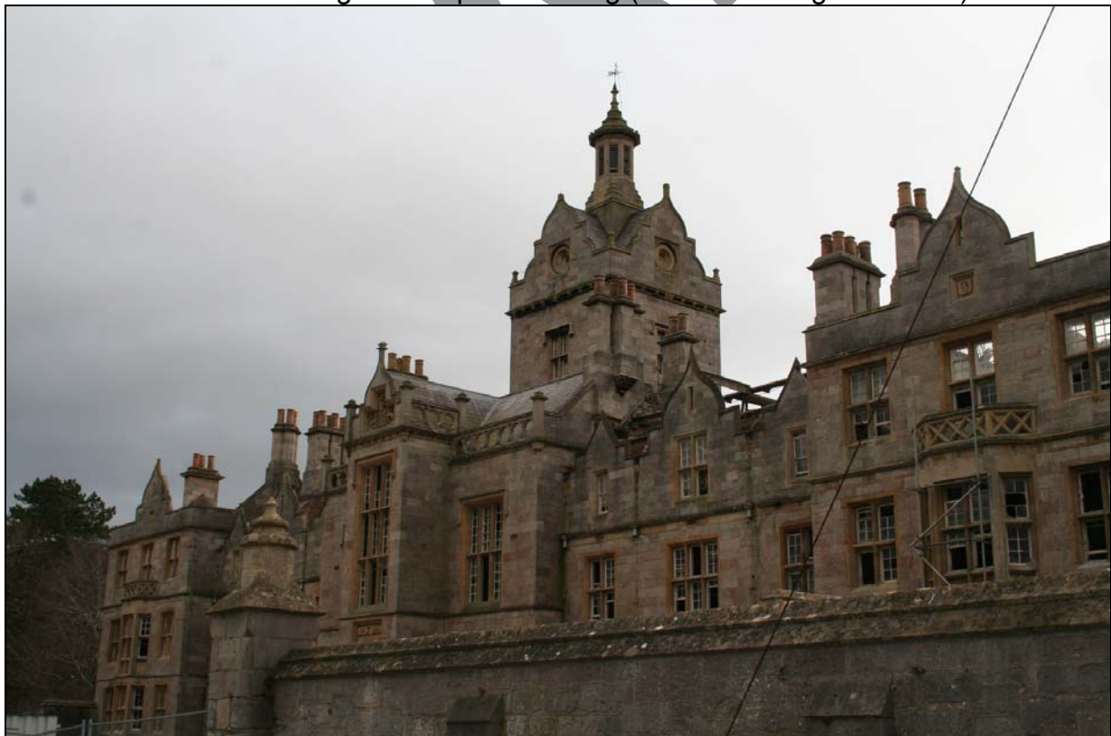
Picture 1: Rear view of original Hospital Building (Listed Building: Grade II*)
